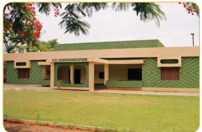
A picture of the 'Kalyanamandapam' equipped with all facilities dedicated to the services of the people of Shreeramnagar for performing social functions
